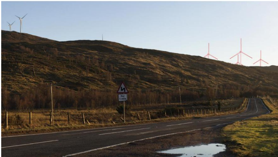
View from A87 north of site
